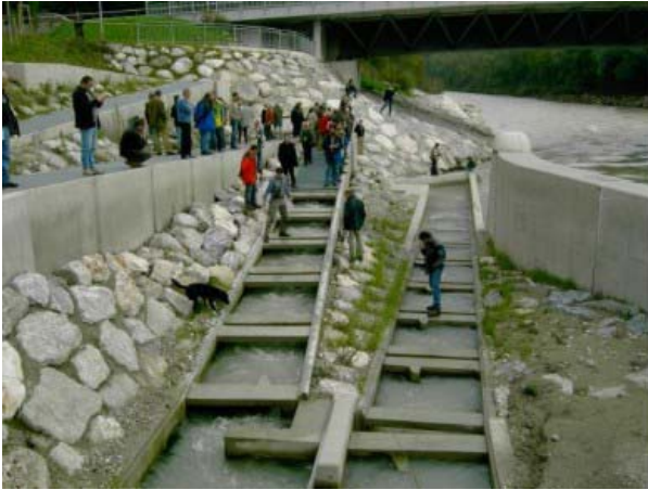
Figure 3: Two types of functioning fish passes – the more natural- like bypass channel is more costly in this case but provides useful additional spawning ground.
